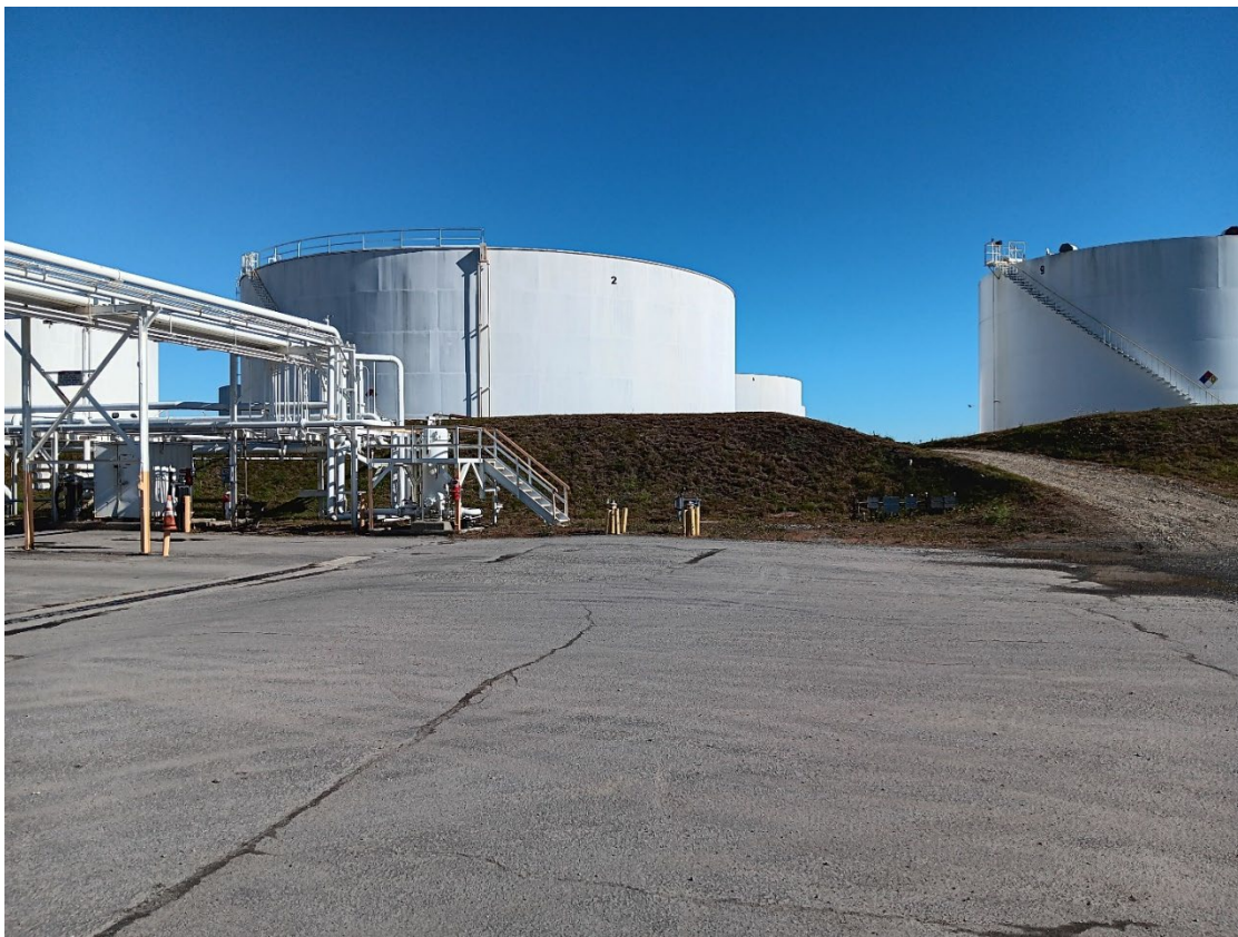
Sunoco, South Portland
