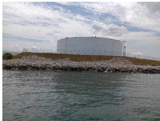
Repairs to tank containment.
